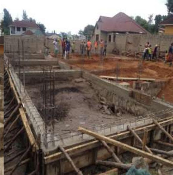
**Column beams:** Columns before for the slab for whole building have been erected. 100% of the work up to the Foundation work has been completed.
